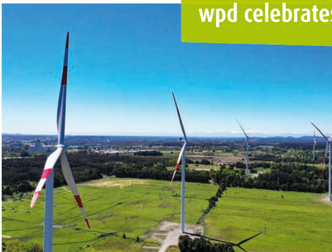
Wind turbines of the Negrete wind farm shortly before commissioning
