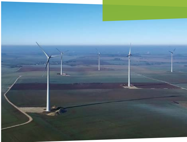
Turbines in the wind farm at Joux-la-Ville commissioned in 2016.
