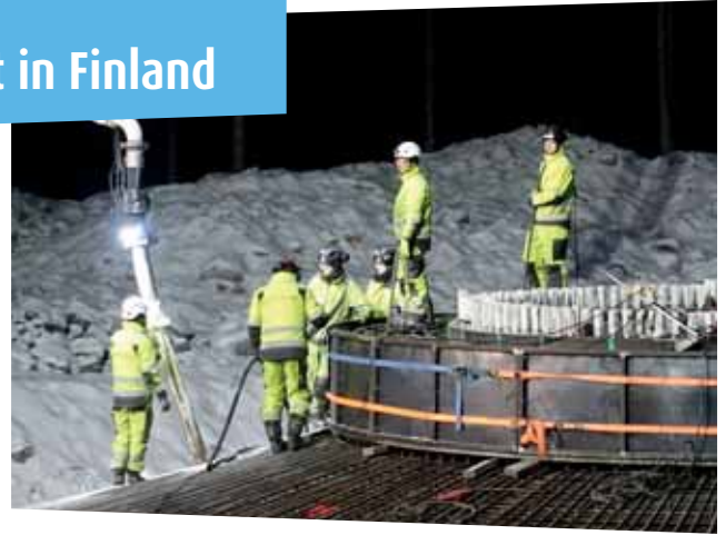
Work on foundations in the Kuuronkallio wind farm
